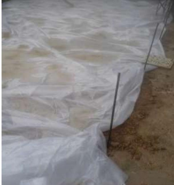
Figure 3: Isolation of simulation model to prevent transmission of water from natural ground.
